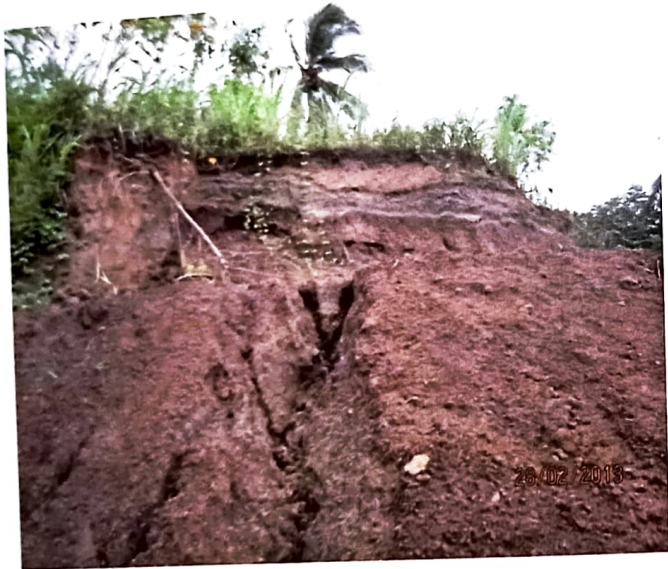
Figure 3.3: Soil Profile shown on a landslide
