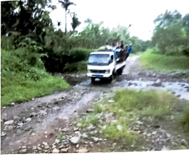
Figure 3.3: Flooded river after a lot of rain fall. Figure 3.4: Lots of rain water run offs damage road infrastructures to rural areas
